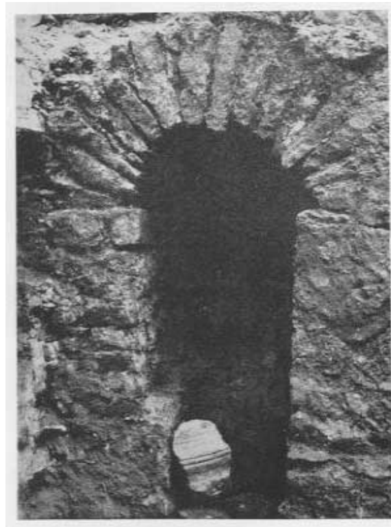
FIG. 28. LINCOLN. SEWER UNDER BAILGATE
